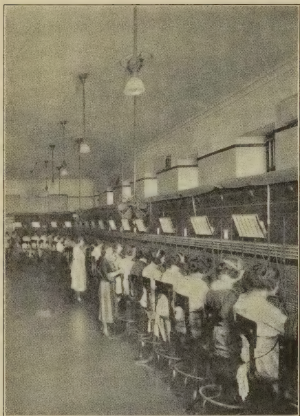
CHelsea TELEPHONE EXCHANGE
